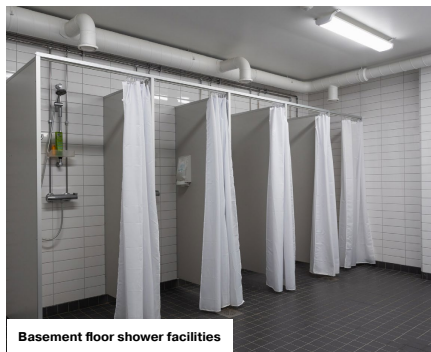
Basement floor shower facilities
