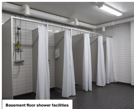
Basement floor shower facilities
